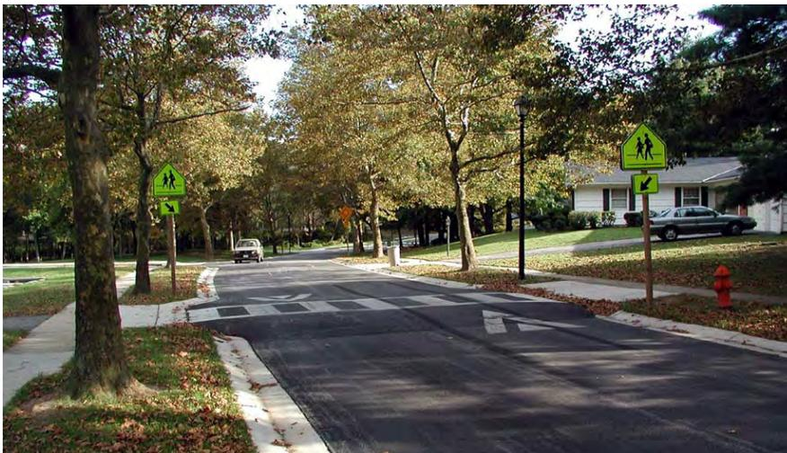
A mid-street raised pedestrian crosswalk, also called a speed table, is appropriate for streets with moderate traffic volume and higher car speeds.
