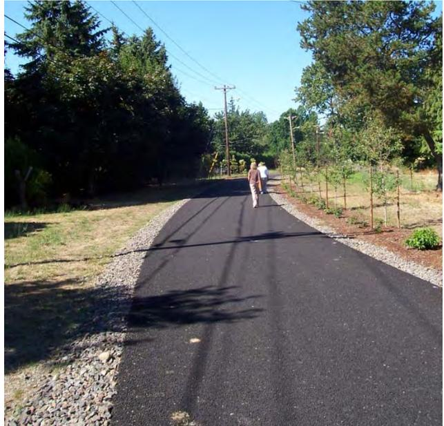
This trail in Gresham, Oregon is an example of a multi-use trail with a pervious asphalt surface that is located on a power line right-of-way.
